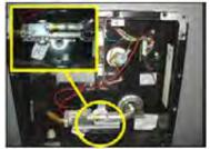
Fig 1: Water heater drain plug
