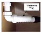
escape into the RV interior. The waterless trap can be unscrewed from the water lines. A label has been placed near the location of the waste valve that reads as follows:
